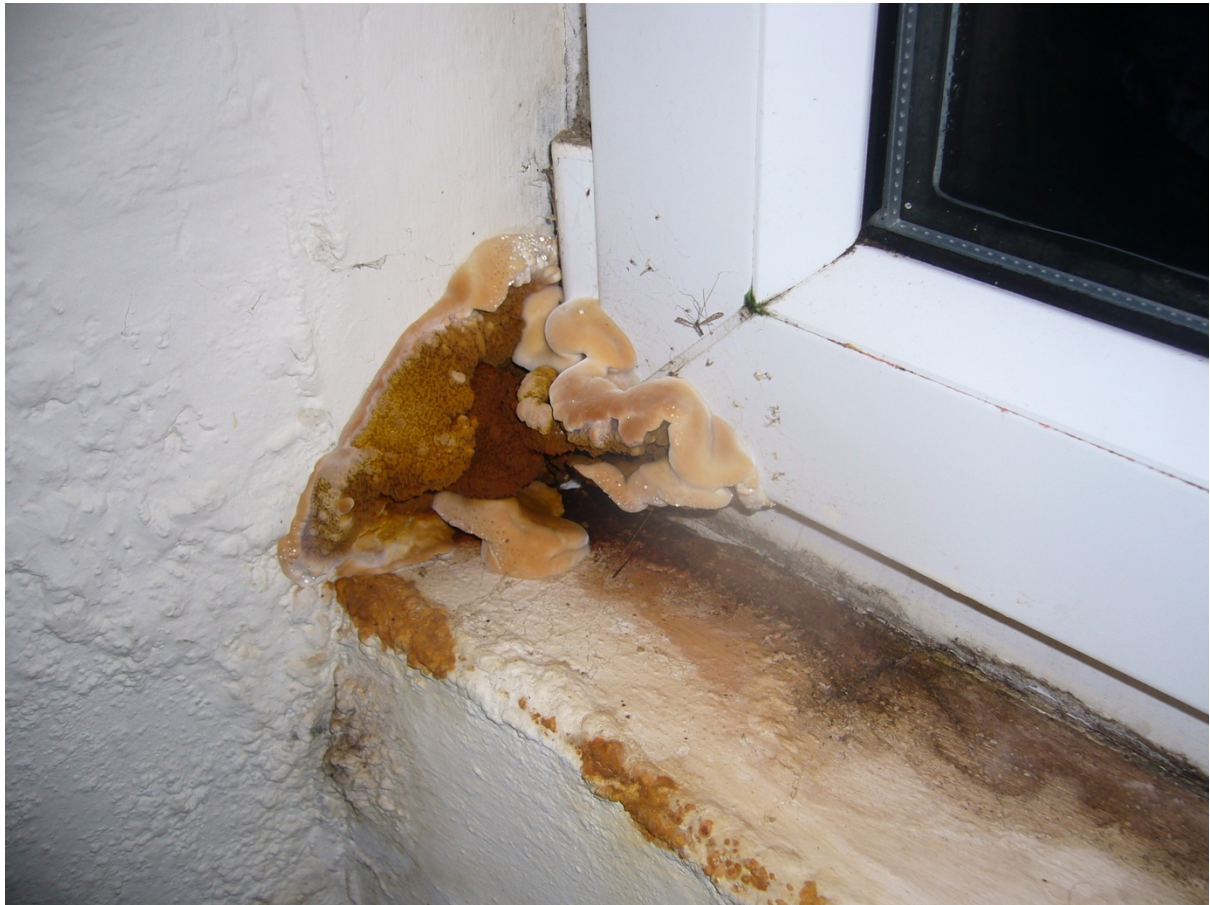
Photo: Dry rot, landing window 25/10/08
