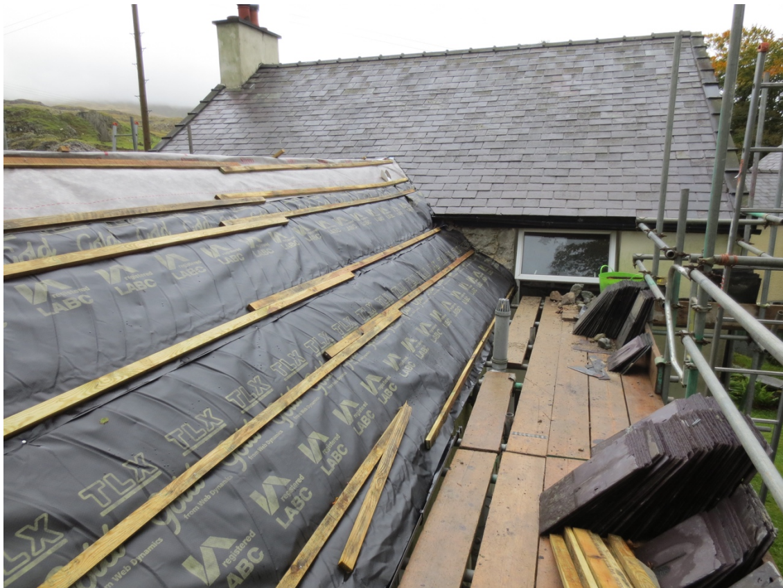
West side new roof with breathable felt and insulation.
