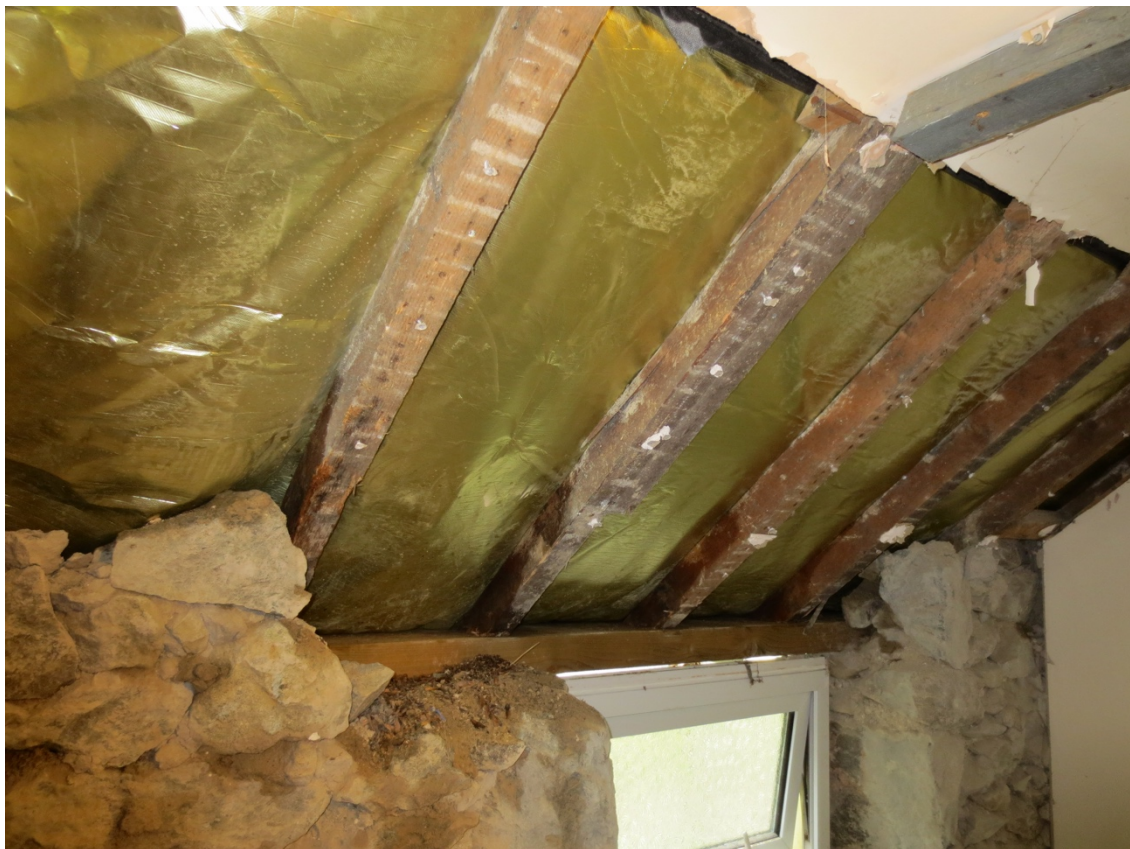
New wall plate and roof insulation above toilet.
