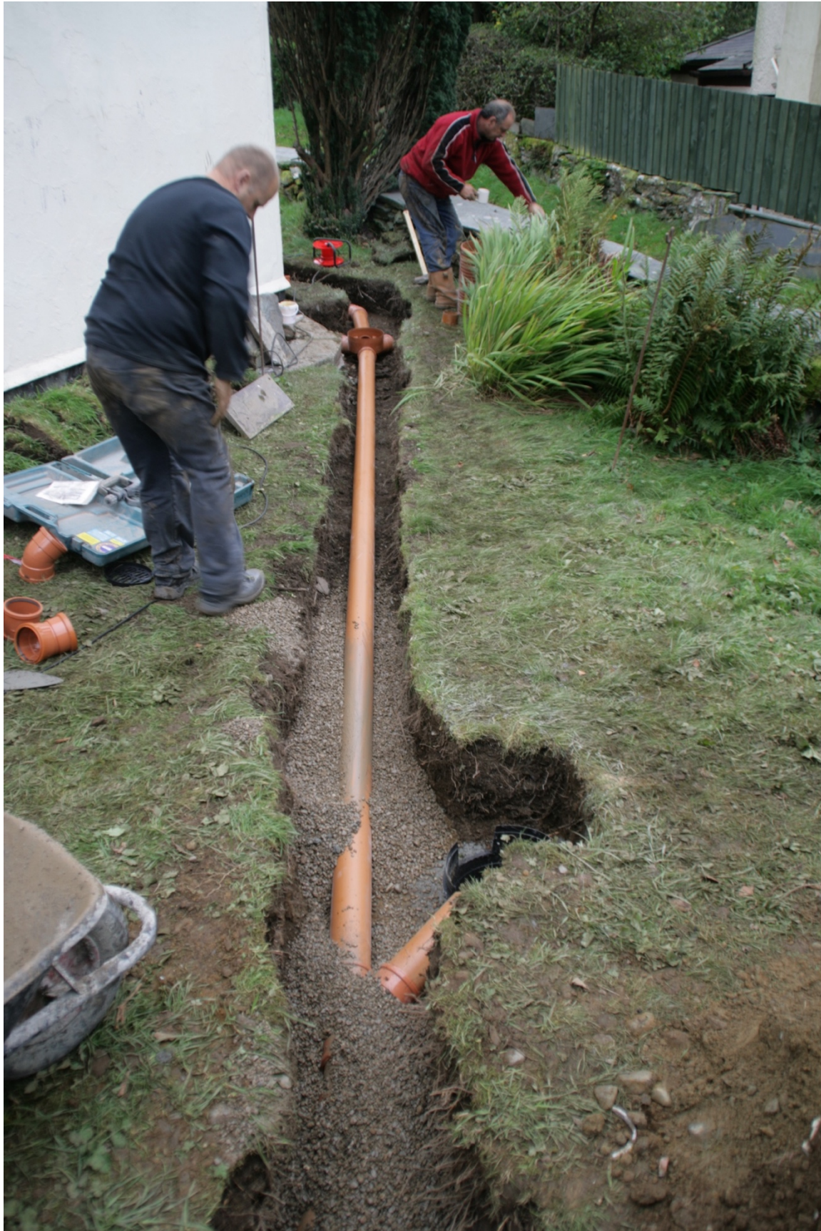
New drain, ground water solids trap, and access branch in SW corner of hut. September 2011.
