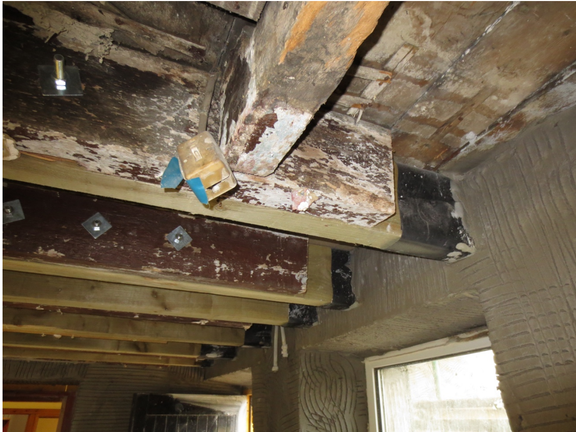
Replacement joist ends (protected) over back room door and window
