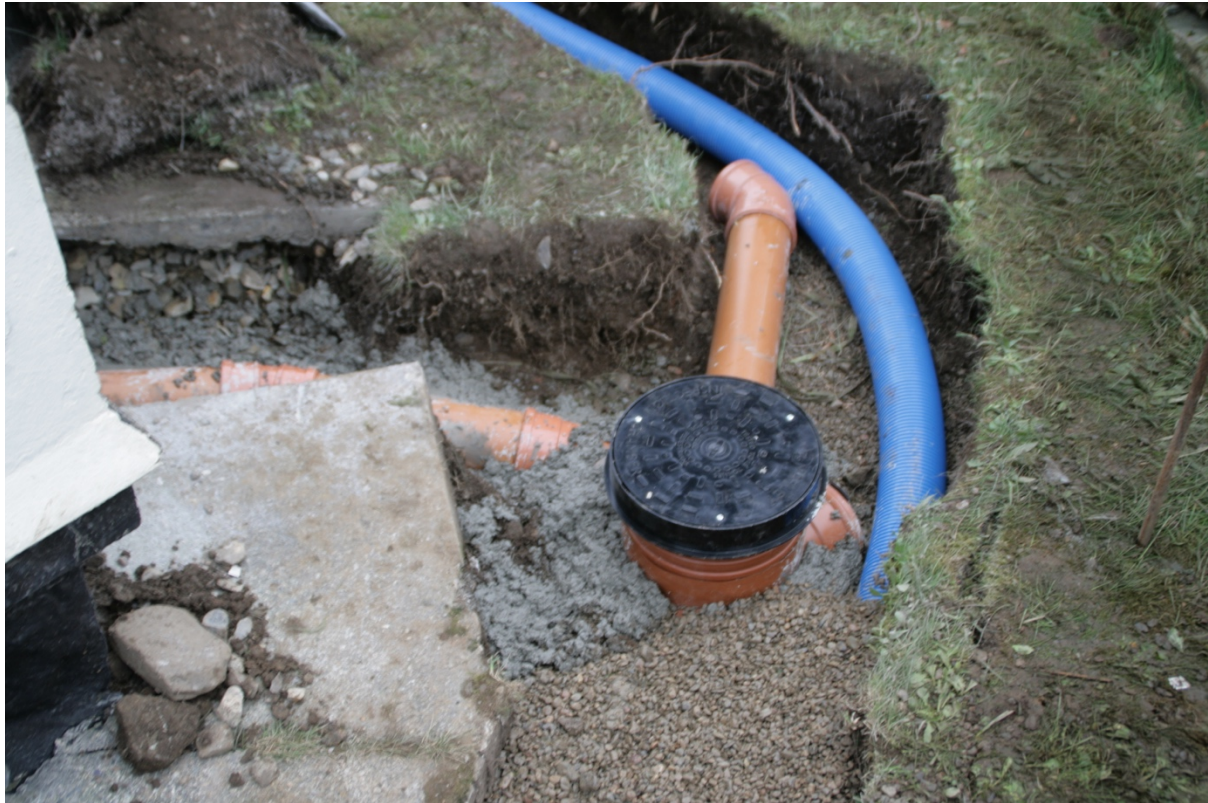
Access branch and ground water perforated pipe at SW corner. September 2011.
