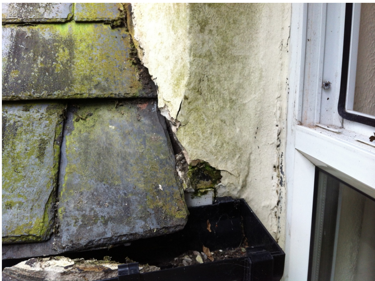
Extension roof, west (Y Garn) side showing poor seal.
