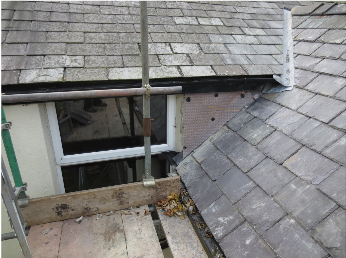
New lead soakers and protective cladding east side.
