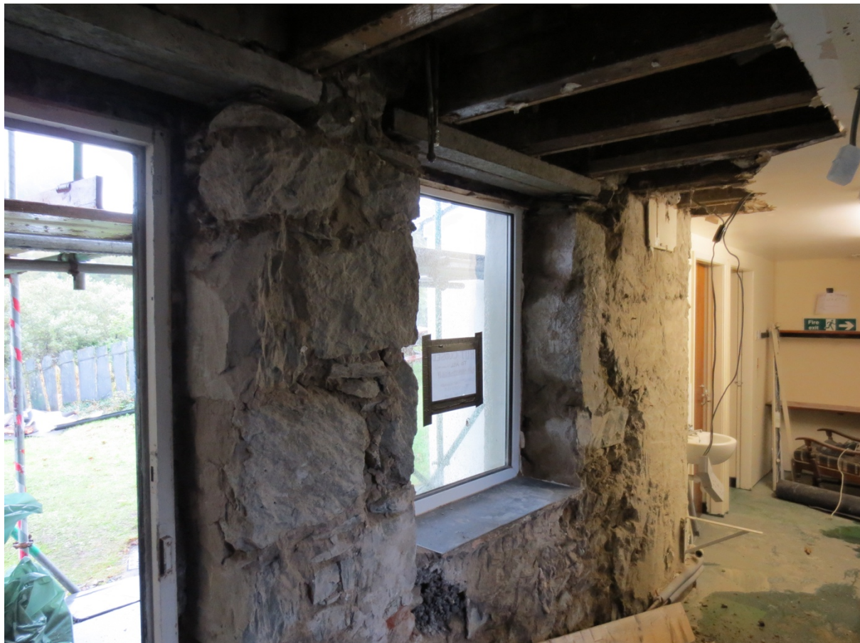
New Concrete lintels over back room door and window, walls stripped.
