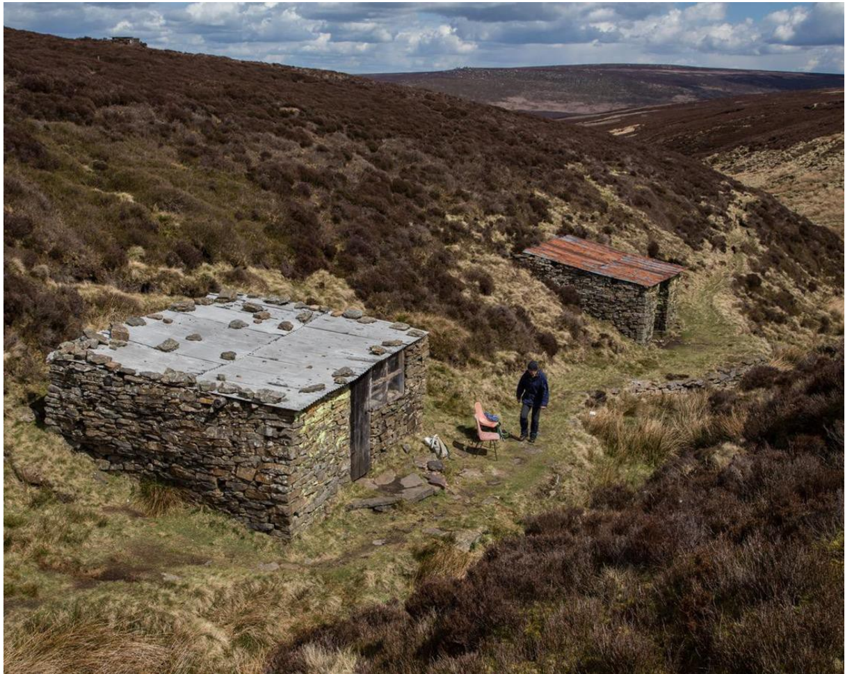
The Lower Small Clough Cabins, the planned location for the bivvy for Saturday, 3rd July. Brian West carrying a quality control inspection
