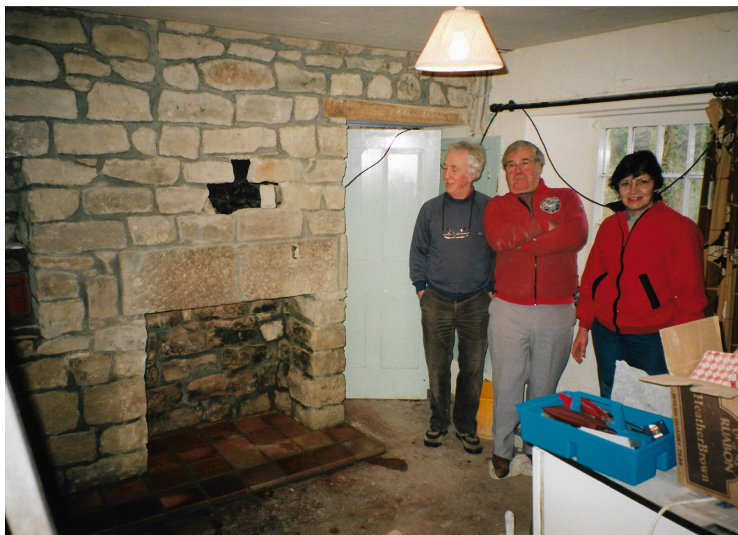
Dave Weston, John Shreeve and Janet admiring the work in progress.
